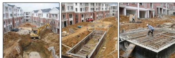
Fig. 4. Excavation, formwork, and casting the storage tank
