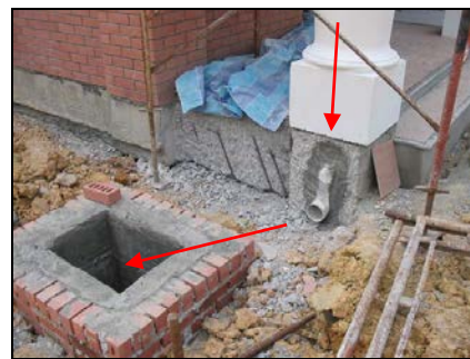
Fig. 3. The collection sump under construction
