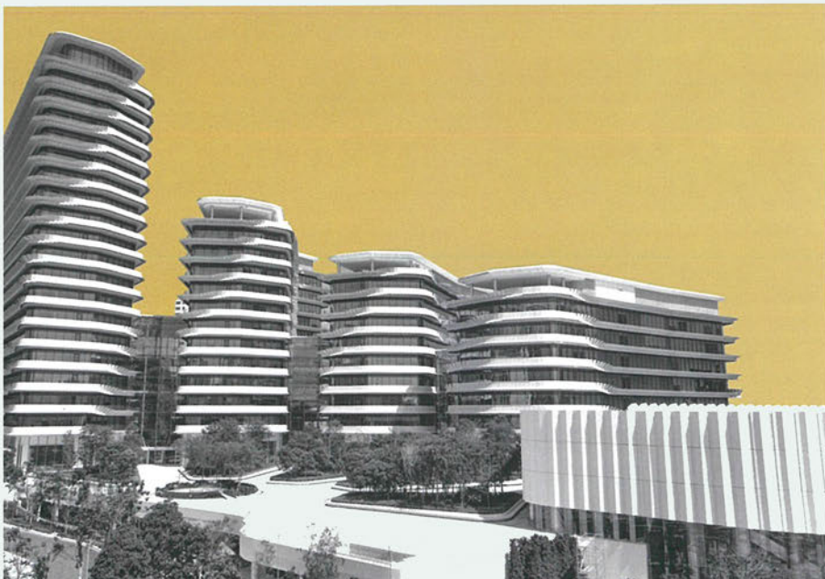
TNB Platinum by Neuforamation Architects in collaboration with Woods Bagot
